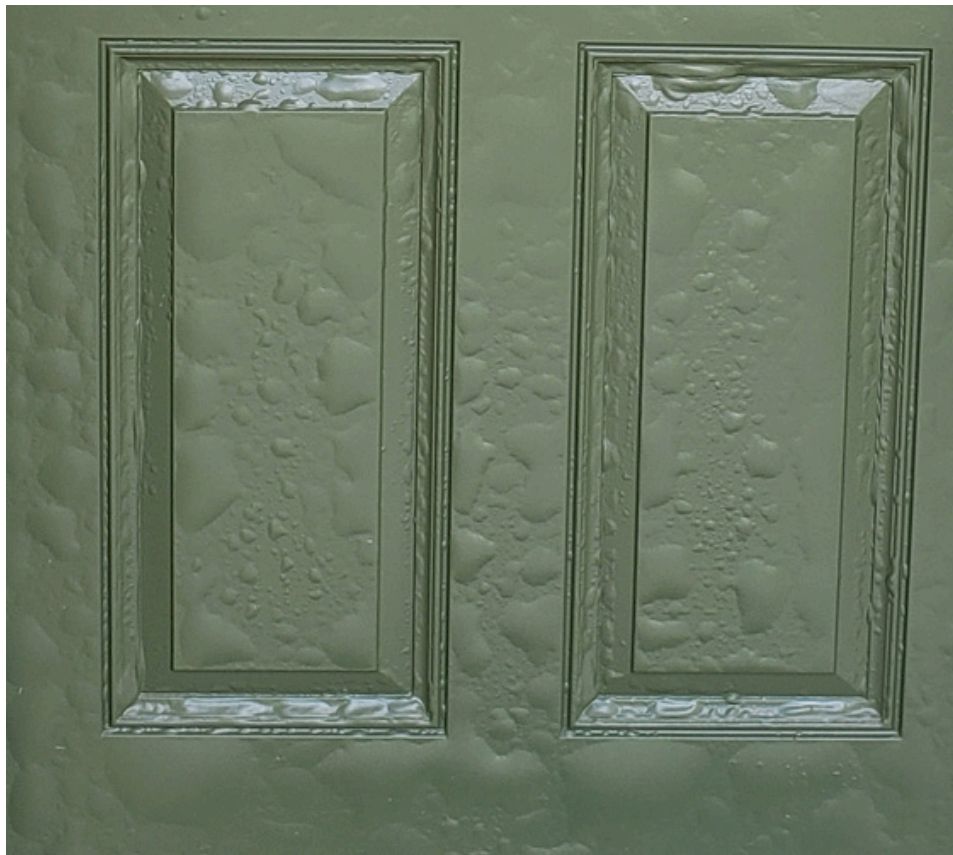
Severe out-gassing blisters on previously painted door.
